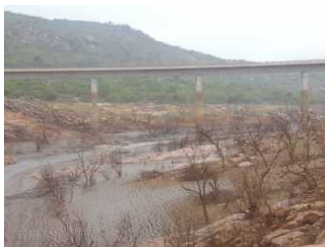
Picture 3: Water level severely decreased at Maguga Dam
