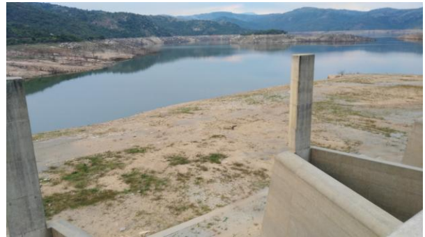
Picture 2: Maguga dam levels
