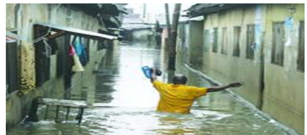
Plate 1: Submerged buildings in a Lagos suburb after Sunday's rainfall that claimed many lives.
