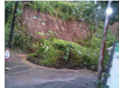
Figure 4 Landslide near Mirabeau, St. Andrew's
